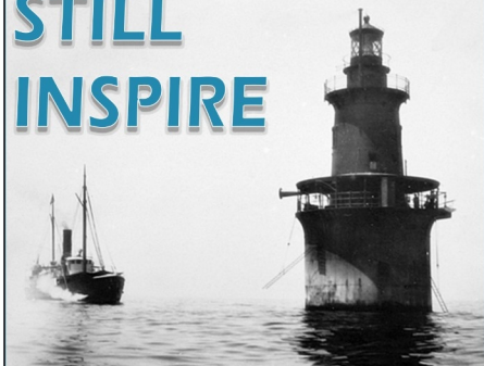
The Sabine Bank Lighthouse
